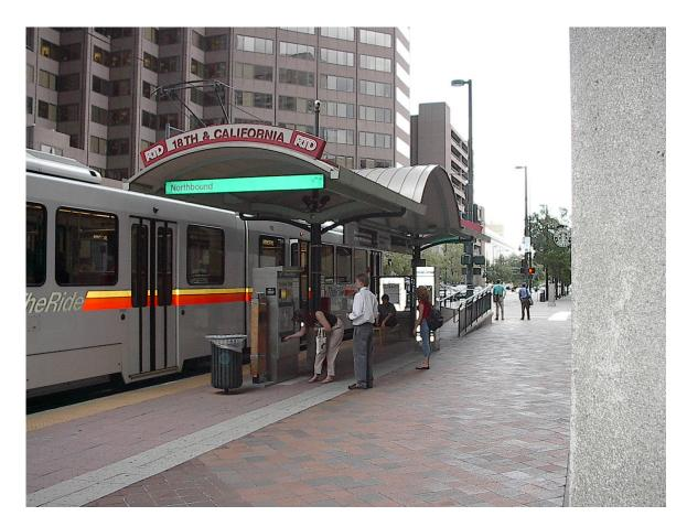
The photo above shows a typical station in downtown Denver where the platform is integrated with the sidewalk. Note that since the Denver LRVs are not true low floor cars (they have steps inside the cars) there is a need for a ramp to provide handicapped access to the head end of the train. It is intended that low floor LRVs for the SE line would be fully accessible and this type of facility would not be required. Overall the station platform amenities are very modest.
